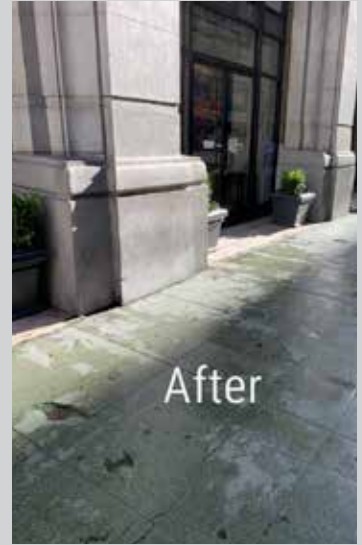
Vandalism in front of our station (after).
